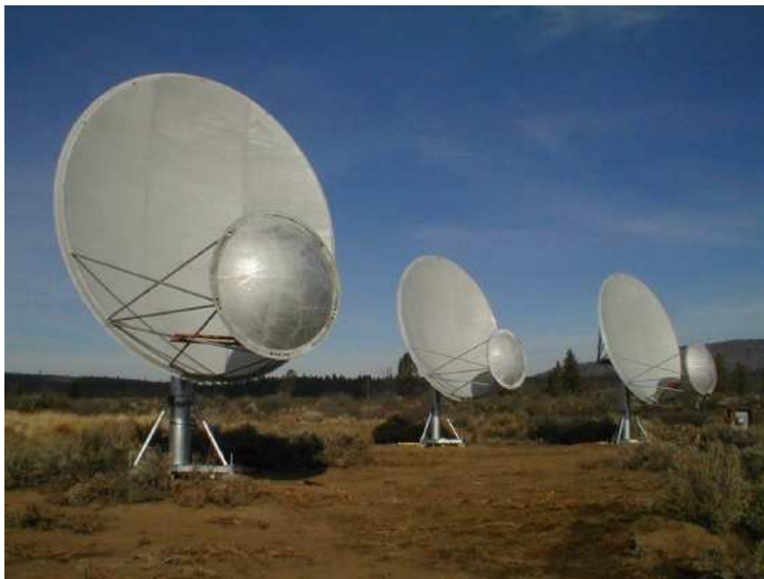
Figure B.1 — First three 6.1m offset-paraboloid antennas of the Allen Telescope Array in Hat Creek, CA.
